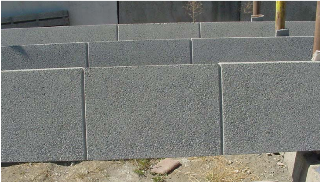
Figure 7. Exposed aggregate after blasting building panels at the large station. The underlying aggregate is clearly visible and the surface appears to have been roughened.
