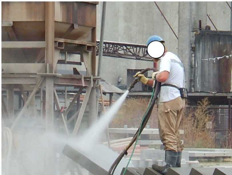
Figure 8. At the small station, the worker performs wet abrasive blasting on fire exit stairs. The bin for filling the abrasive blasting pot is in the background on the left. The aggregate is barely visible.
