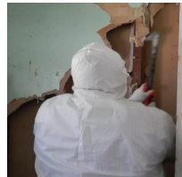
Worker wearing protective gear when removing mold.
