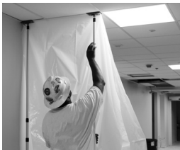
Worker establishing a containment area during an ICRA training class.
