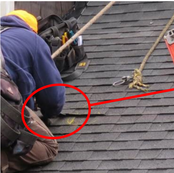
Fig. 2 Lifting up composite shingles to inset connection plates
