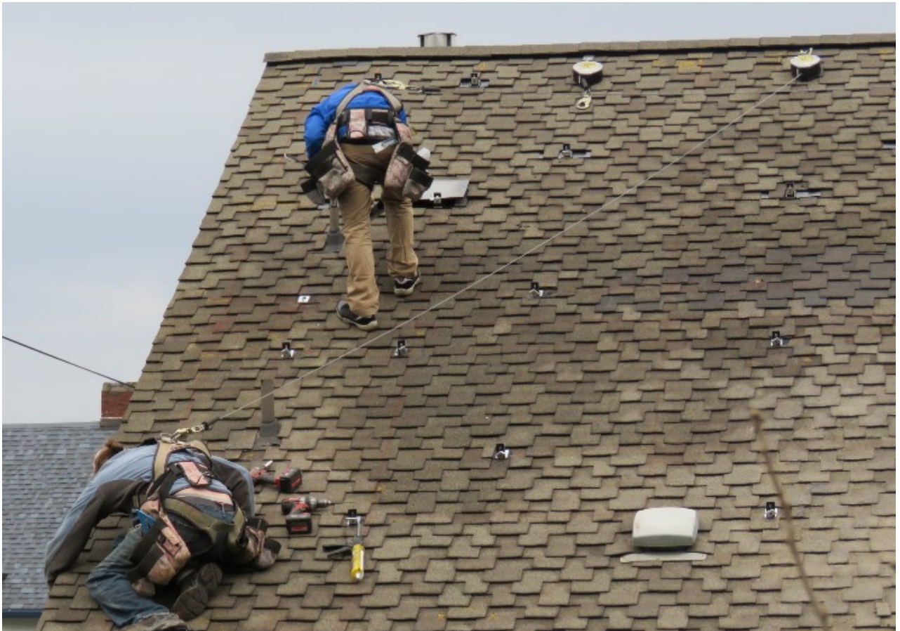
Fig. 3 Installing connection brackets on a sloped roof.
