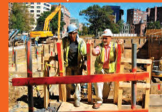
AUGUST Early construction: Sheeting and shoring process
