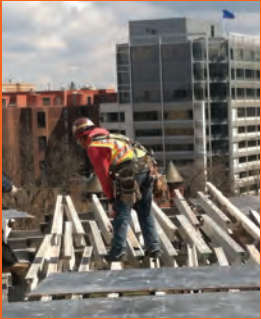
MARCH Roofing phase
