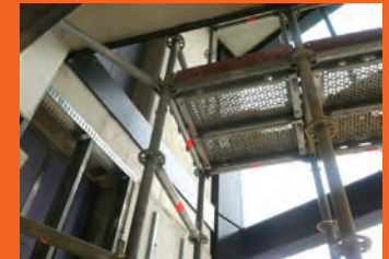
SEPTEMBER Interior rough-in continues
