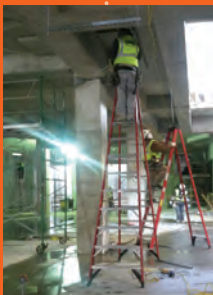
MARCH Concrete placement phase
