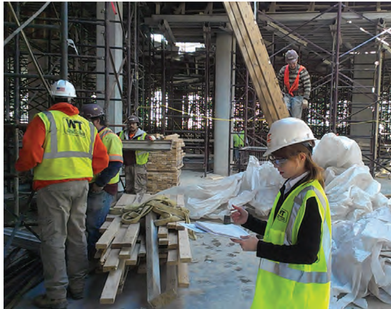
Researchers visited the construction site 38 times between April 2013 and March 2014.
