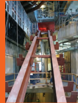
AUGUST Interior rough-in phase
