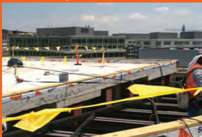
AUGUST Roofing continues
