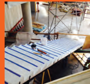
NOVEMBER Interior finishes phase
