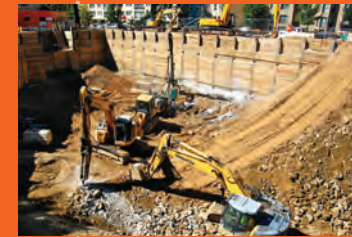
JULY Early construction: Creating basement levels
