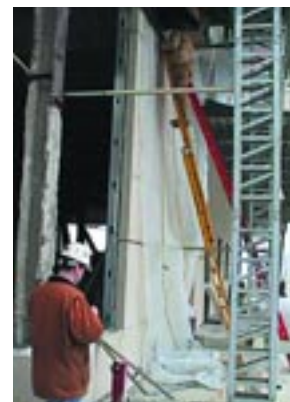
A Fall-Safe auditor checks a worksite in West Virginia. The bottom of the worker's ladder should be further out from the wall.
