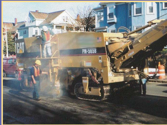
Members of a milling crew from Laborers local 22 and Operators local 4 work in Cambridge, Mass., in 2000. (Courtesy Harvard School of Public Health)
