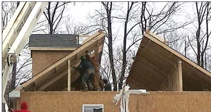
Raising the roof
