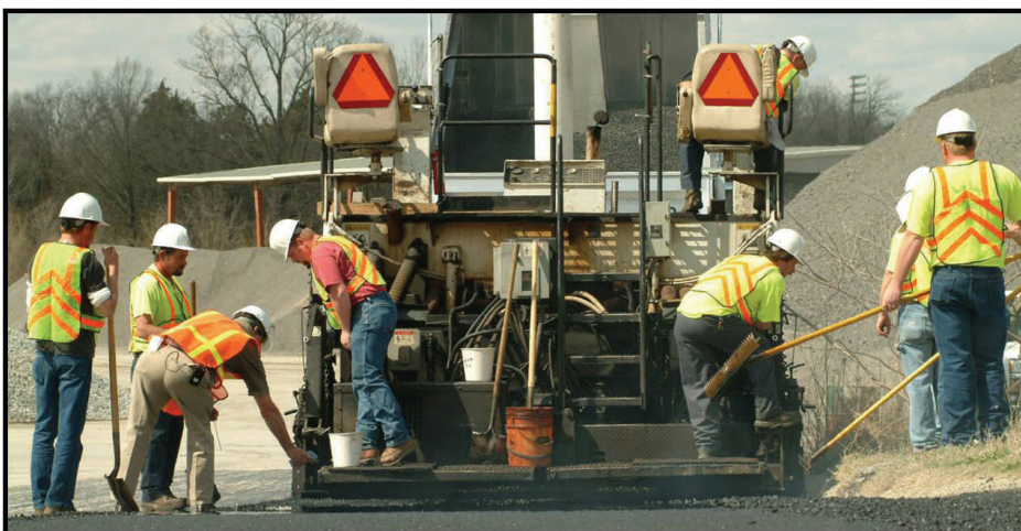
Above: Warm-Mix Asphalt (Photo: NAPA)
