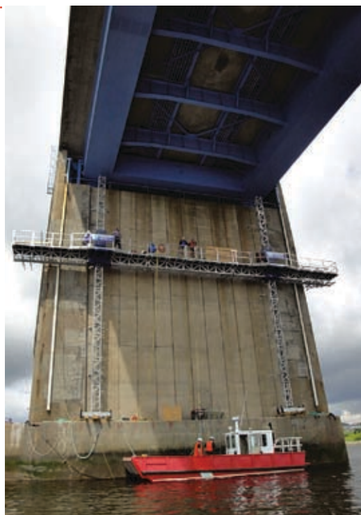
Use of twin masts on the Saint John Harbor Bridge Pier in Saint John, New Brunswick, Canada, illustrates the flexibility and small footprint of mast climbers. Photo courtesy of Klimer Manufacturing, Inc.
