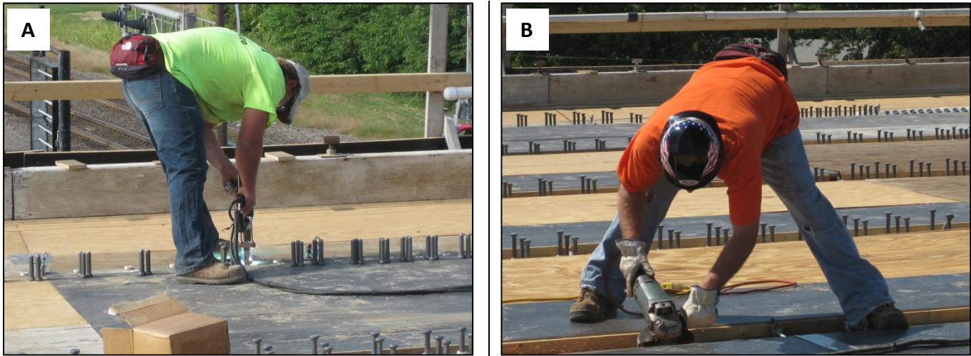
Figure 2: A – stud welding using traditional equipment; B – preparing weld locations with an angle grinder.
