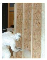
Figure 36. JobCorp student using a soy-based spray foam.
