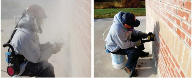
Figure 39. Tuck-pointing without controls
