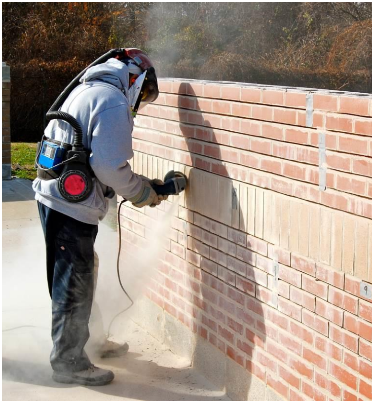
Figure 2. Bosch grinder without tuckpointing LEV system.
