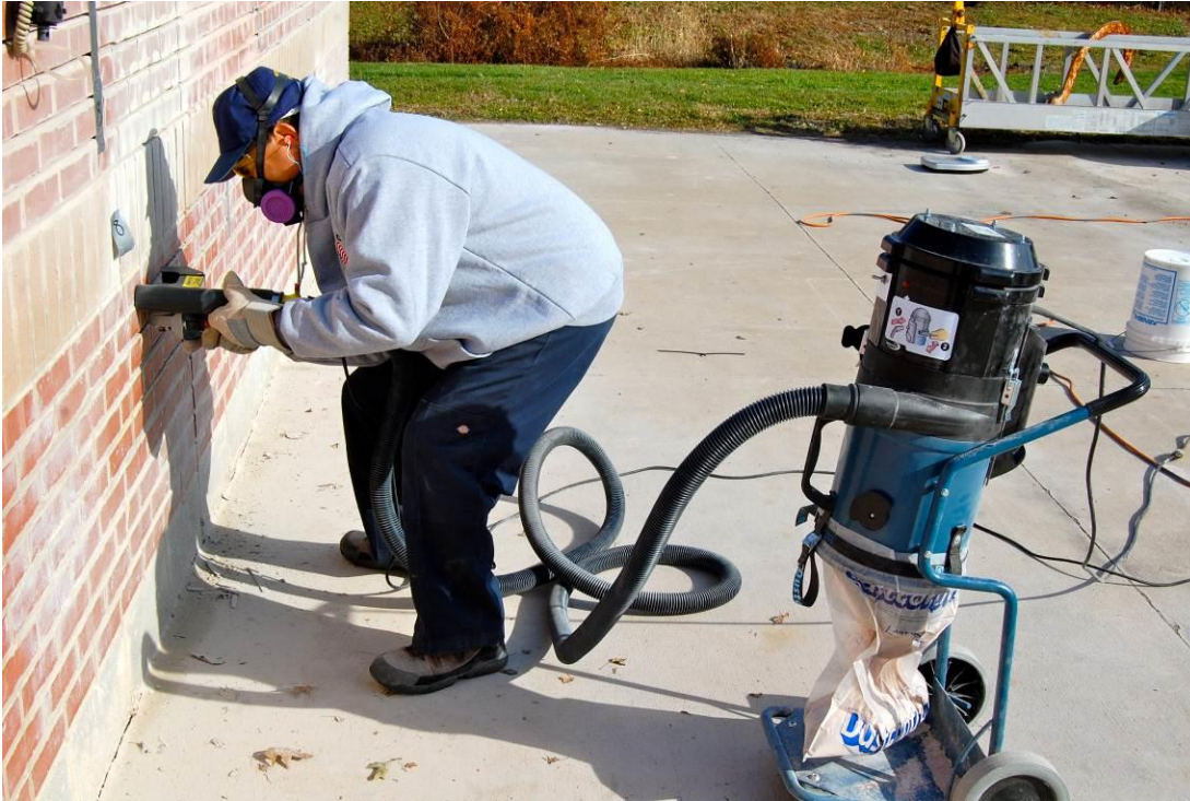
Figure 3: Bosch Grinder with LEV System
