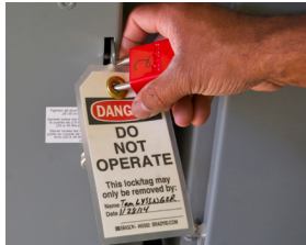
A machine being locked and tagged out.
