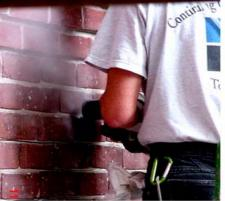
B. When the gap between the mortar and the exhaust take-off is too large, mortar debris escapes between the exhaust take-off and the mortar. In the picture on the right, the grinder take-off is not flush against the wall and a dust plume is faintly visible between the exhaust take-off and the wall.
