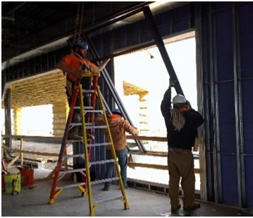
6d-Frame Installation/Lifting
