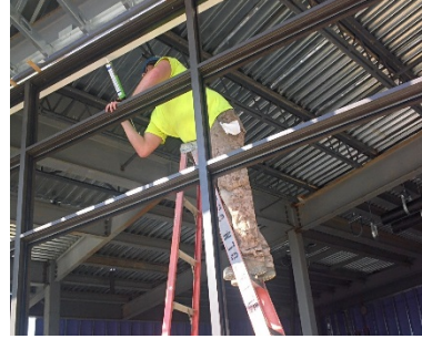
9c- Apply /Push the Caulk Bead
