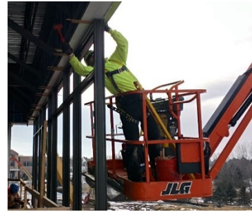
6f- Storefront Installation/Shimming
