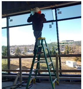
7e- MMH / Placing
