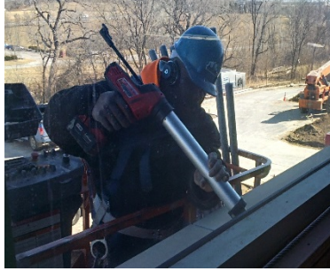
9b- Apply /Push the Caulk Bead
