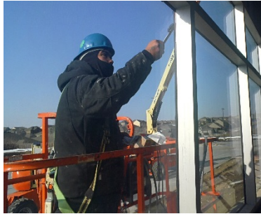
9e- Smooth the Bead with Finishing Tool
