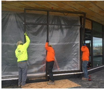
6e- Frame Installation/Placing
