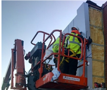
8e- MMH / Placing
