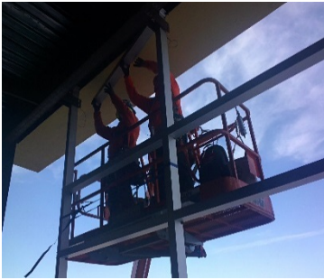
6a- Curtain Wall Installation
