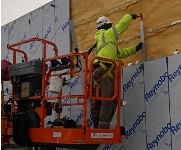
8d- Panel Installation
