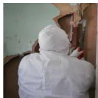
Worker wearing protective gear when removing mold.
