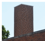
Faux chimney conceals 15 panel antennas
