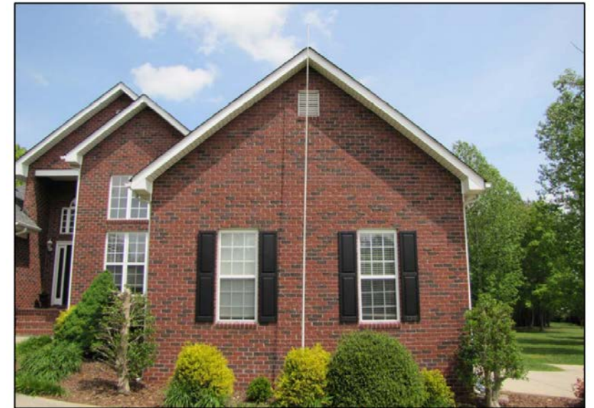
Photo 1. Roof pitch of the garage was determined to be 10/12 (Photo courtesy of NCDOL/OSH)
