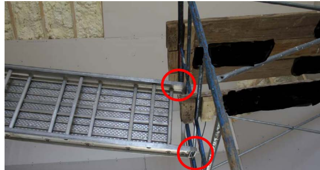
Figure 3. Position of the plank after the accident. Note the lack of attaching hooks (circled)
