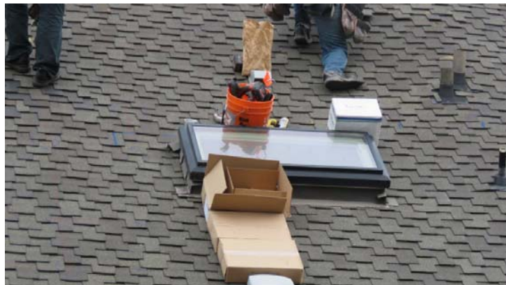
Figure 7. Using Skylight to Hold up Installation Tools and Materials (Picture taken by Chung Ho on 11/17/2016 at Case Study 1)
