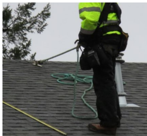
Fig. 11 This project installed Guardian bull ring anchors along the roof ridge.
