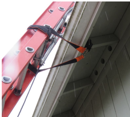
Fig. 13 Ladder stabilization device
