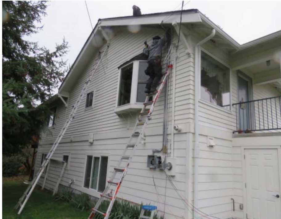
Figure 11. Running the Wire for Solar System (Picture taken by Chung Ho on 12/02/2016 at Project 3)
