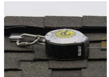
Figure 3. Fall Protection System (Picture taken by Chung Ho on Nov. 17, 2016 at Case Study 1)
