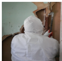
Worker wearing protective gear when removing mold.
