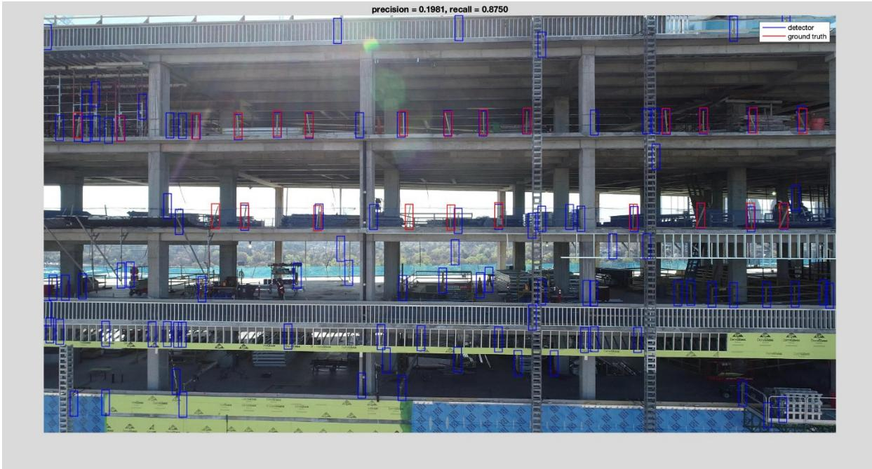
**Figure 11: Visualizations of the guardrail detections using linear SVM**
