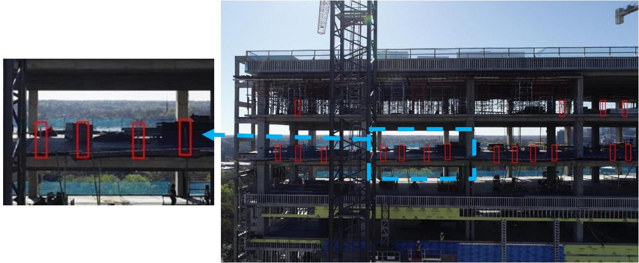
**Figure 2: Visualization of the labeled bounding box of guardrails**
