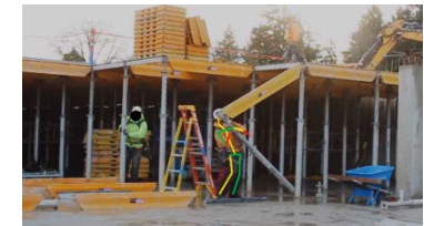
Plumb a shoring post
