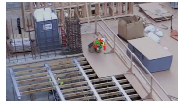
Nail a sheathing panel to supporting members
