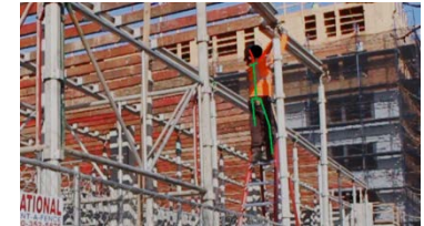
Lift a main beam
