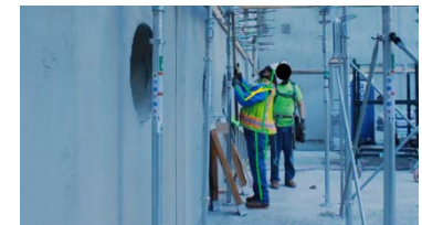
Inspect with a level
