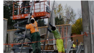
Hold a shoring post in place
