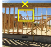
Framer fell from rim joist (x) above window opening to floor deck.
