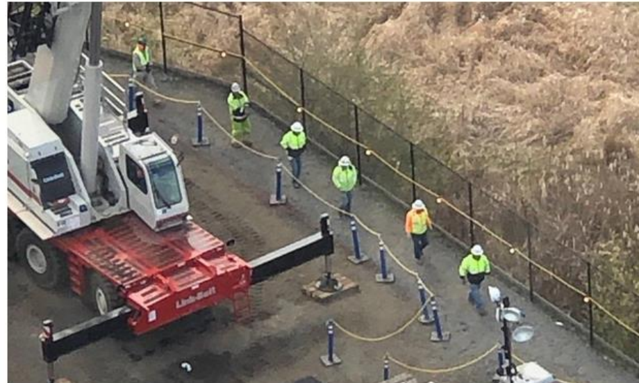
Using physical distancing on construction site.
