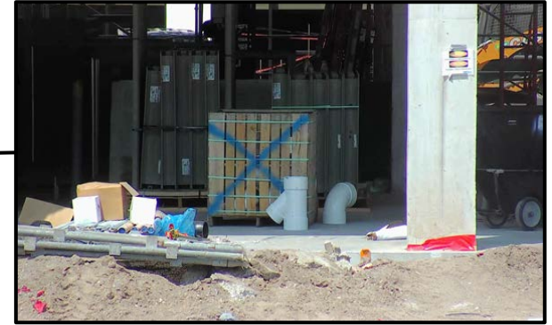
Tripping Hazard: Improper indoor housekeeping
