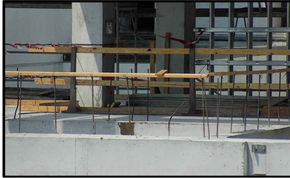
Fall Hazard: Improper installation of guardrails in some indoor openings
