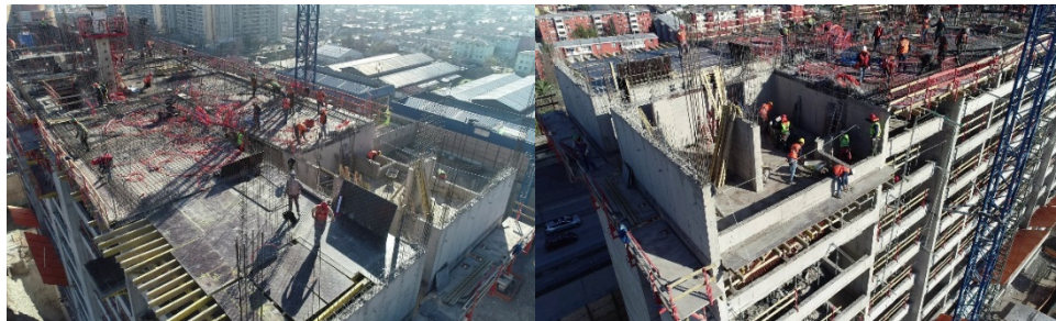
Lack of guardrails
