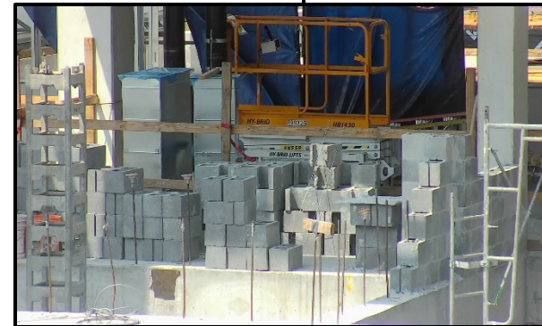
Struck-by Hazard: Improper storage of material located in indoor areas
