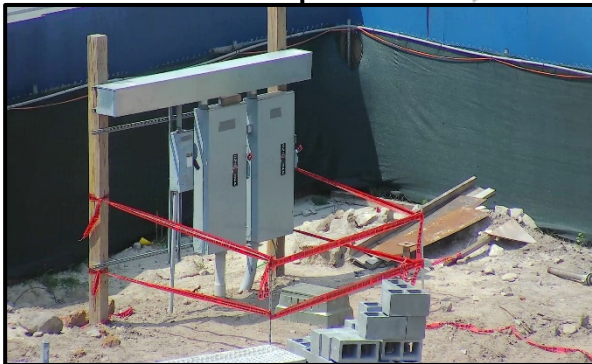
Electrical Hazard: Improper warning signs around the electrical panel
