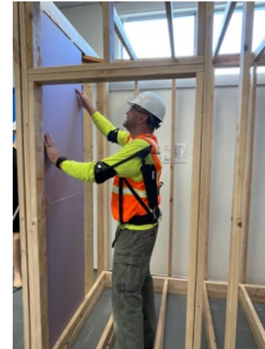
Drywall Installation
