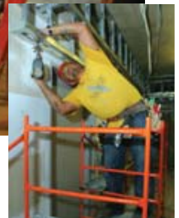
Dr. Rempel's overhead drilling device, above, means a more comfortable posture, reduced muscle fatigue, and decreased hand vibration, unlike the traditional method (at right).
