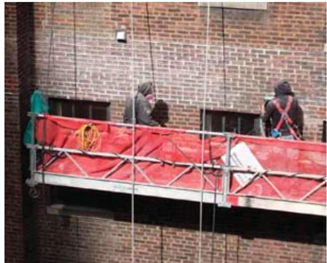
Silica Dust: Above, workers are tuck-pointing, or removing mortar between bricks, without a control device. Below, use of a dust control device significantly reduces hazardous dust.
