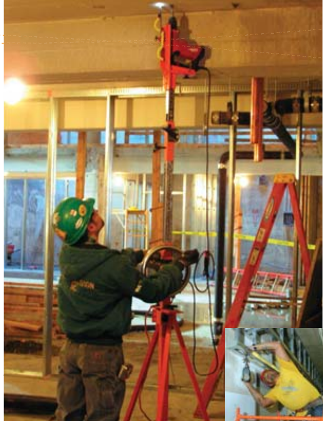
Dr. Rempel's overhead drilling device, above, means a more comfortable posture, reduced muscle fatigue, and decreased hand vibration, unlike the traditional method (at right).
