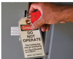
A machine being locked and tagged out.
