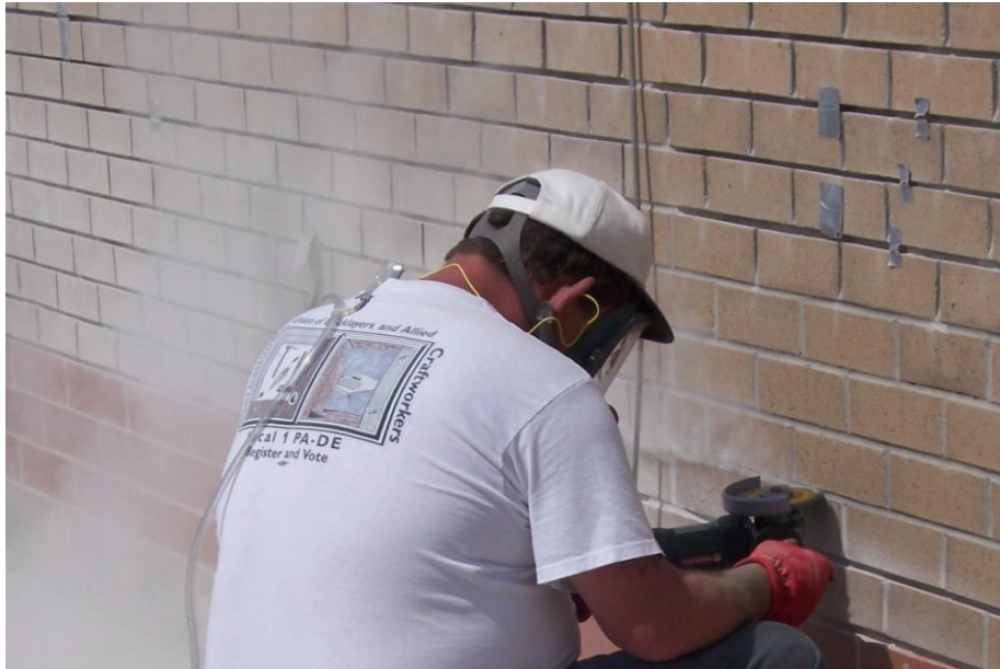
Figure 2. Metabo grinder without tuckpointing LEV system
