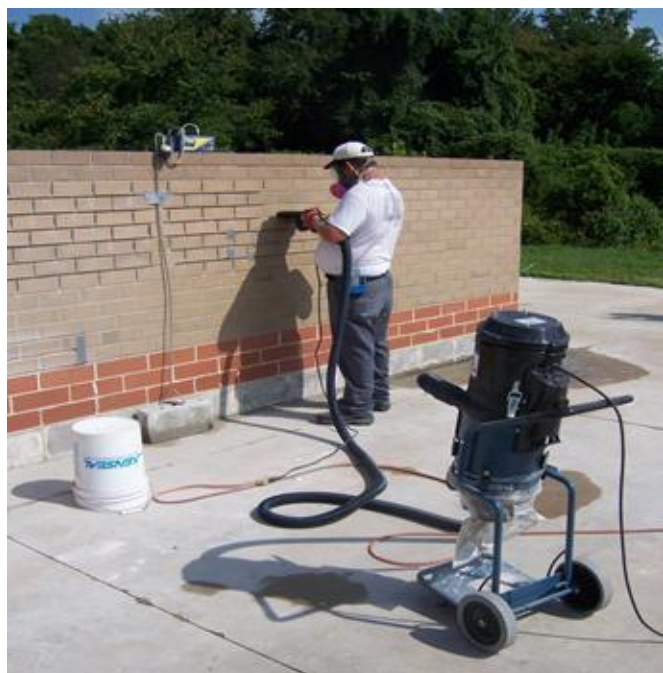
Figure 3. Metabo grinder with Dust Director shroud and DustControl 2900c vacuum
