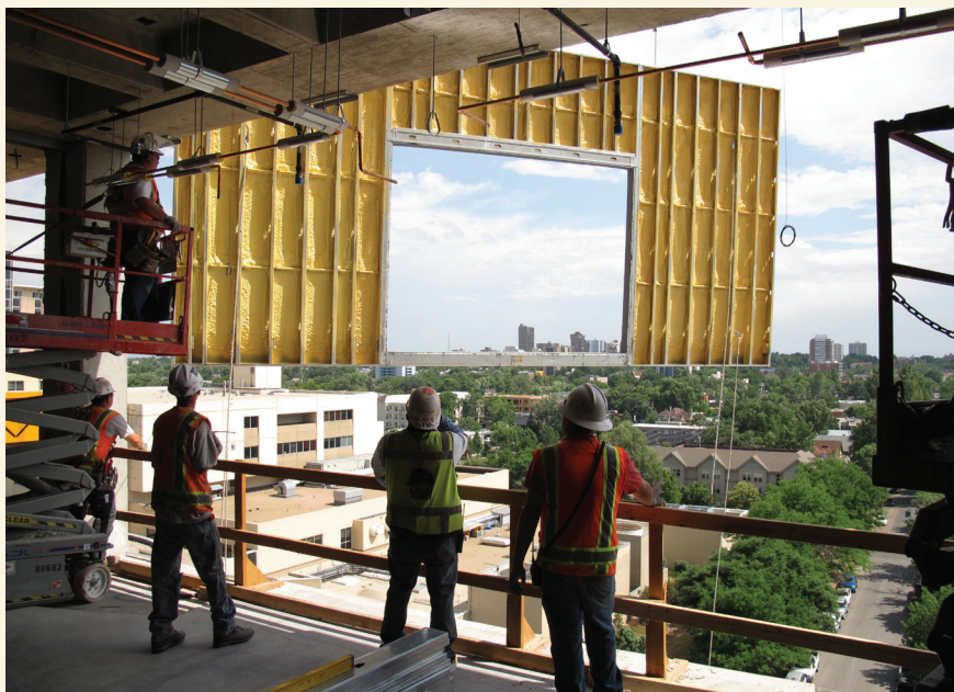
Installation of a prefabricated exterior wall panel.
