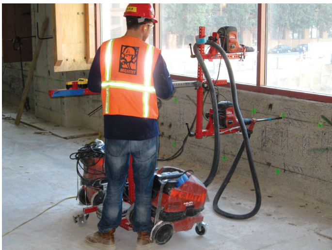
Laborer at a San Francisco site using drilling jig set up for 2 drills but only drilling with one. Concrete dust is captured during drilling with a new hollow bit system.
