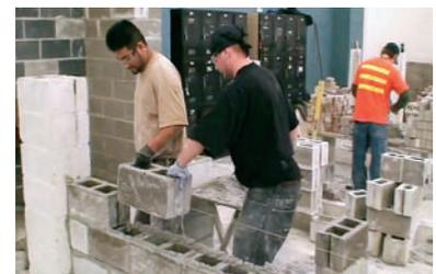
Workers use a two-person team lift technique to reduce stress of lifting and twisting.
