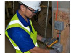
Worker testing a circuit to ensure that it is de-energized
