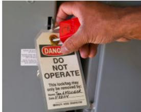
A machine being locked and tagged out.
