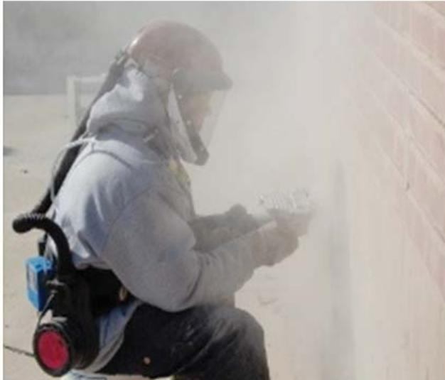
Figure 39. Tuck-pointing without controls
