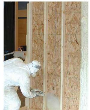
Figure 36. JobCorp student using a soy-based spray foam.
