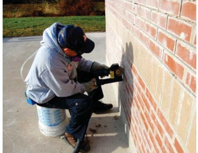
Figure 40. Tuck-pointing with controls
