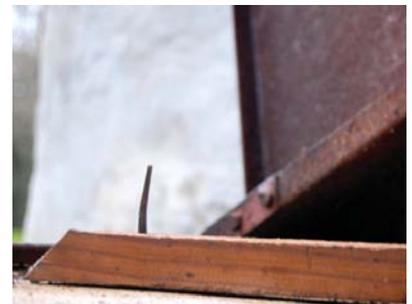
Figure 22. Nail protruding from wood.
