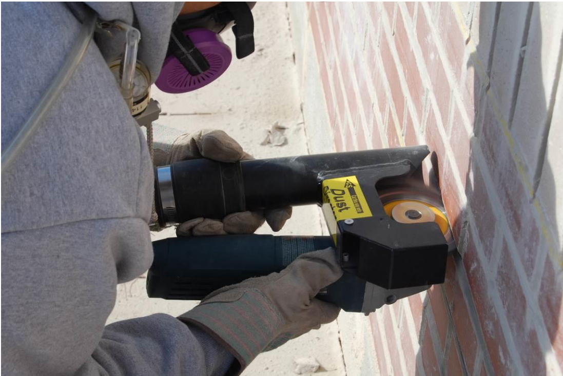
Figure 1. Bosch grinder with Dust Director shroud
