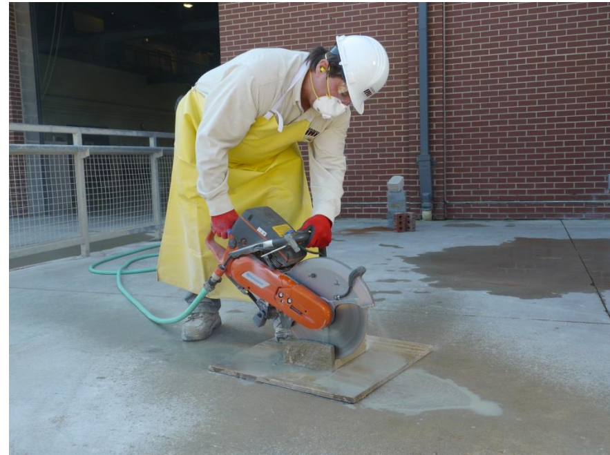
Photo courtesy of the International Masonry Institute & OSHA
