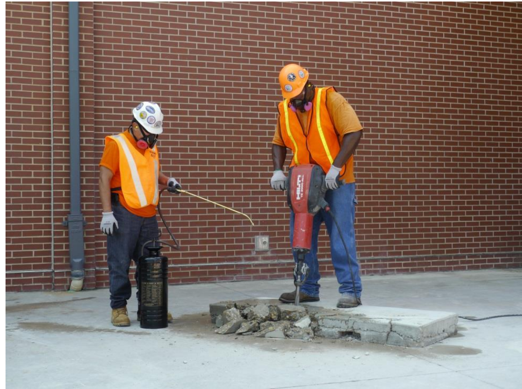
Photo courtesy of the International Masonry Institute & OSHA
