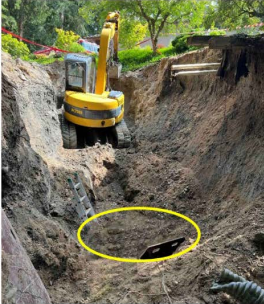
Photos 2 and 3. Two views of the incident scene. The yellow circles show where workers were in a 5-foot wide, 10-foot deep ditch at the bottom of the trench.
