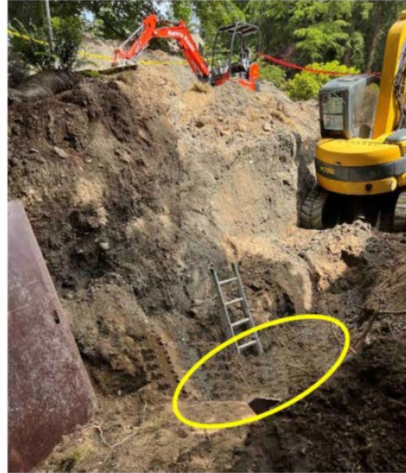
Photos 2 and 3. Two views of the incident scene. The yellow circles show where workers were in a 5-foot wide, 10-foot deep ditch at the bottom of the trench.
