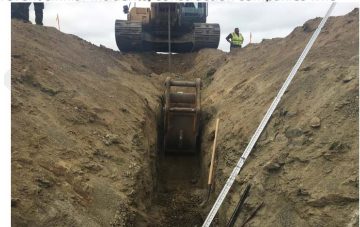
Exhibit 4. Slope and depth of the trench.
