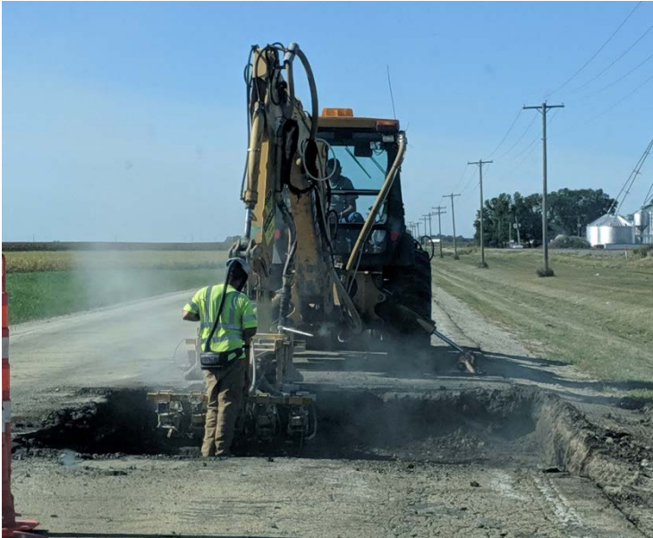
Employee operating drill rig
