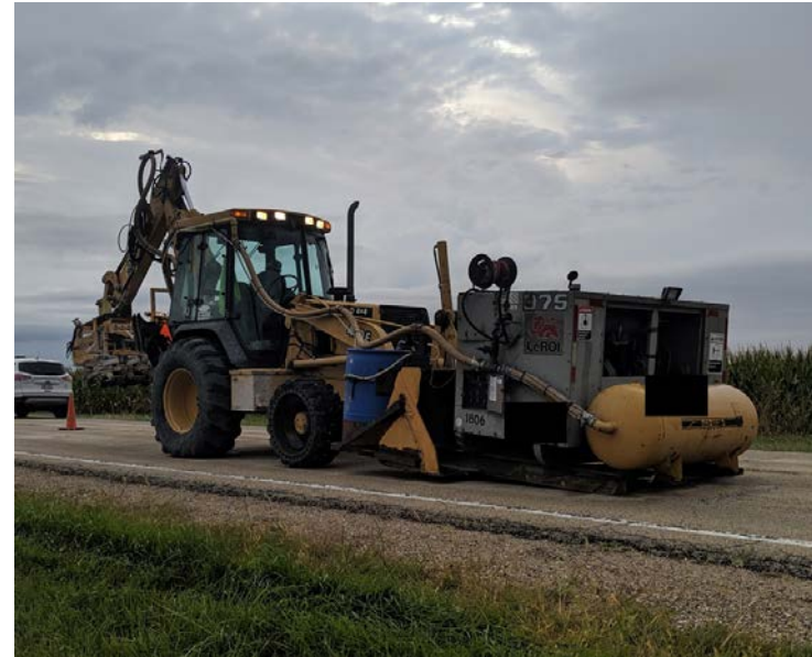
Drill rig is on the arm of the backhoe, Water reservoir on the front bucket
