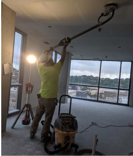
Powered sander connected to HEPA shop vacuum
