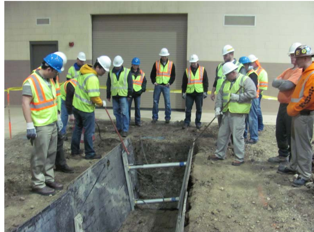
OTI #3010 – Trenching and Excavating Course
