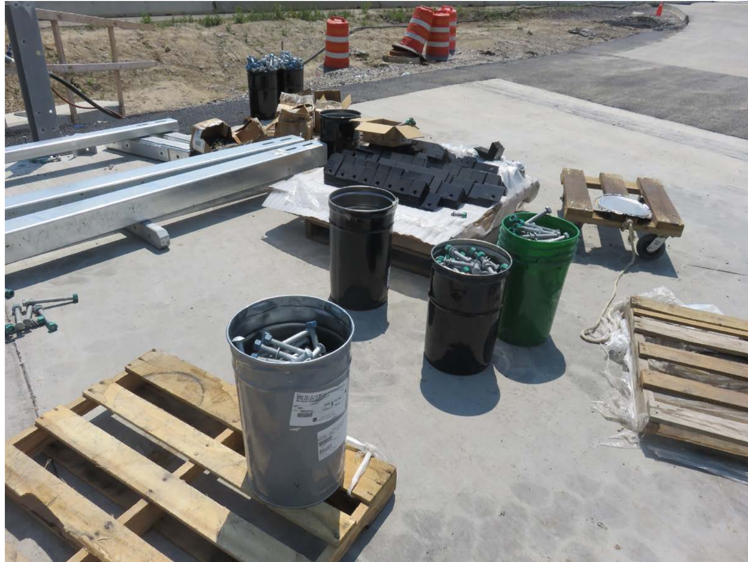
Employee was sorting railing bolts for the roadway barriers
