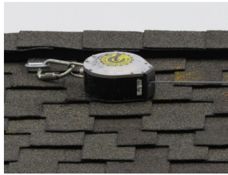
Fig. 10 This project installed Hitchclips along the roof ridge to serve as safety anchors.
