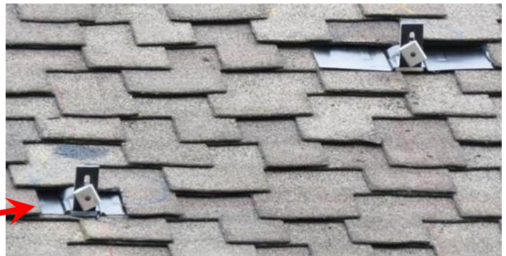
Fig. 2 Lifting up composite shingles to inset connection plates
