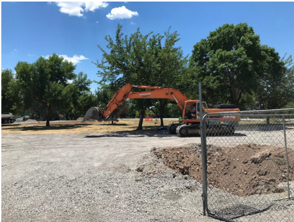
Figure 5 – Salt Lake City sampling location at university family housing construction site.
