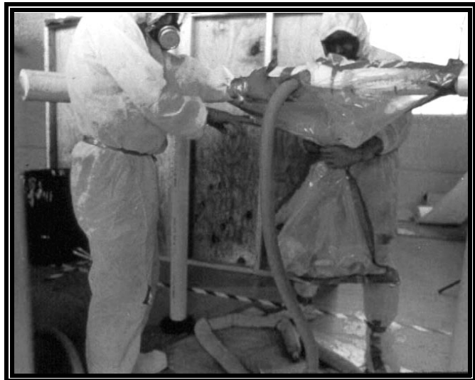
Removing the glovebag after a repair.
