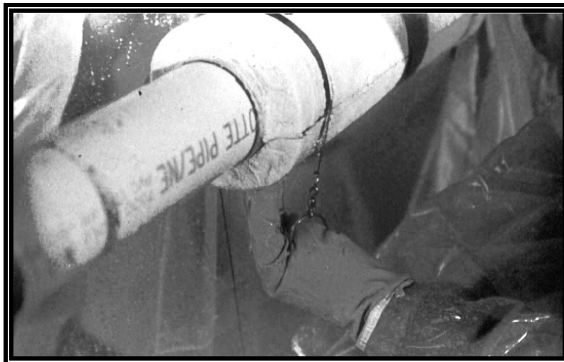
Using a bone-saw to remove pipe covering ACM – in a glovebag
