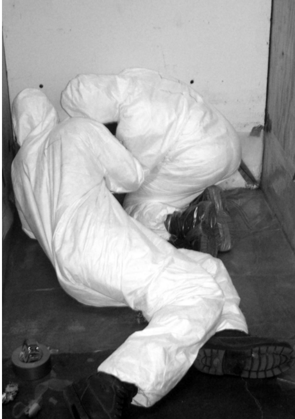
... how to make “hospital corners” while laying floor poly...
