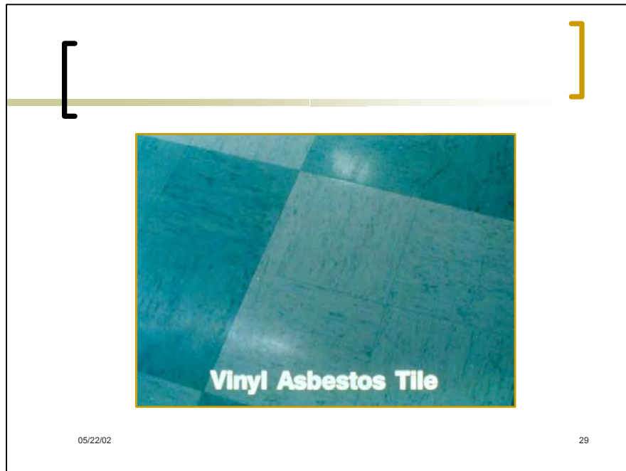
SLIDE #29 (Tray 1 – 95): Vinyl asbestos tile
