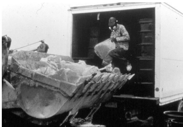
Off-loading bagged ACM waste at a EPA - approved land fill.
