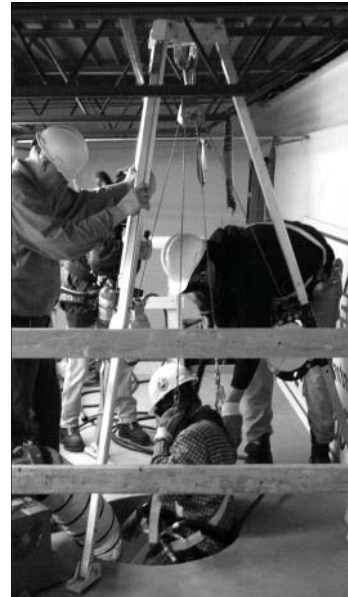
SAR-supplied entrant with 7' tripod, attendant, supervisor, and mechanical ventilation.
