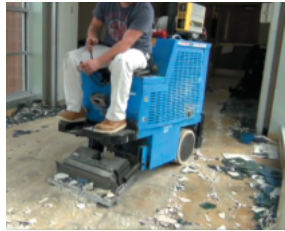
Breaking tile, not backs, can be done with a ride-on floor scraper, the “Terminator.”
