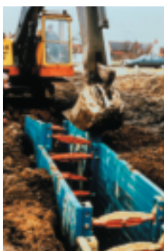
Gallegos' search ended on eLCOSH with this photo showing a poorly installed shield that would not restrict hazardous lateral movement.
