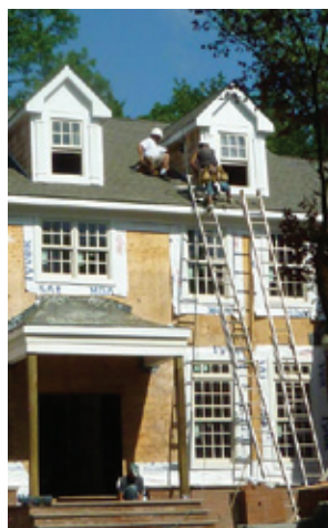
Typical New Jersey residential construction conditions faced by safety liaisons as recorded by project staff. Intervention can save the lives of workers at risk of a fatal fall.
