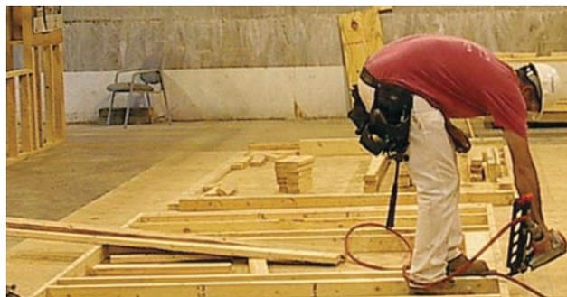
and experience. The data will be used to provide feedback to the International Staple Nail and Tool Association about safety materials included in tool packaging. At the same time, the research team is comparing the productivity of the two types of triggers when used by experienced journeymen.
