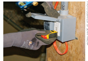
Testing a GFCI outlet to make sure it was wired correctly.
